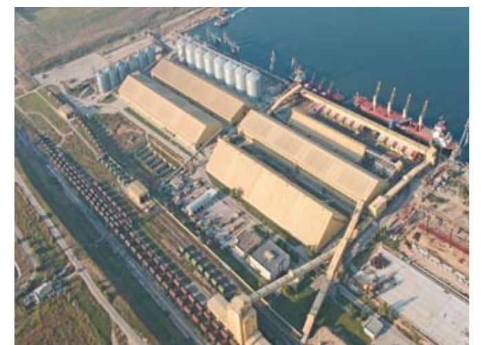
Loading and unloading facilities
